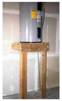
Figure 6: Permanent mitigation - platform hot water heater above BFE.
